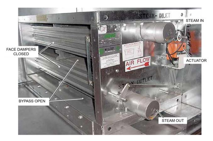
FIGURE 83 - IFB COIL (HORIZONTAL TUBES AVAILABLE WITH STEAM AND HOT WATER)
