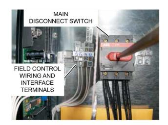
FIGURE 69 - TYPICAL FIELD AND POWER CONNECTIONS
