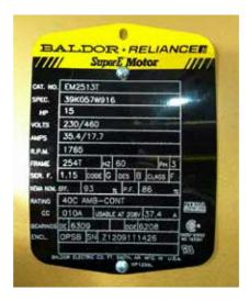
FIGURE 62 - TYPICAL MOTOR DATA/NAME PLATE
