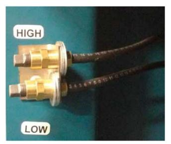
FIGURE 57 - HIGH AND LOW CONNECTIONS FOR AN IN FAN AIR MONITORING SYSTEM
