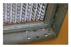
**FIGURE 111 -** CORRECTLY INSTALLED CARTRIDGE FILTER
