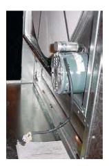
FIGURE 65 - TYPICAL POWER WIRING OF ENERGY RECOVERY WHEEL
