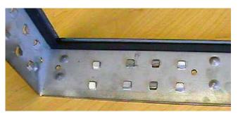
FIGURE 114 - CORRECT USE OF KNOCKOUTS
