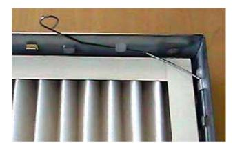
FIGURE 108 - FULLY INSTALLED FILTER
