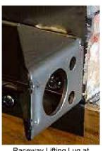
Raceway Lifting Lug at Shipping Split Before Assembly
