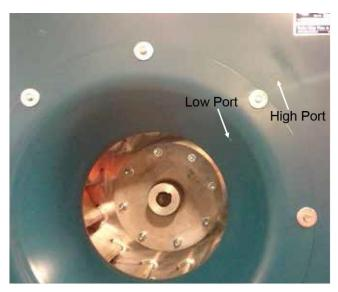
FIGURE 58 - PORT LOCATIONS FOR FAN MOUNT-ED AIR MONITORING SYSTEM
