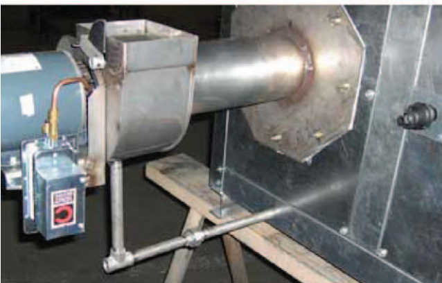
FIGURE 24 - SET ID FAN DAMPER
