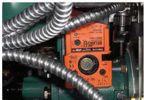
FIGURE 28 - DAMPER ACTUATOR
