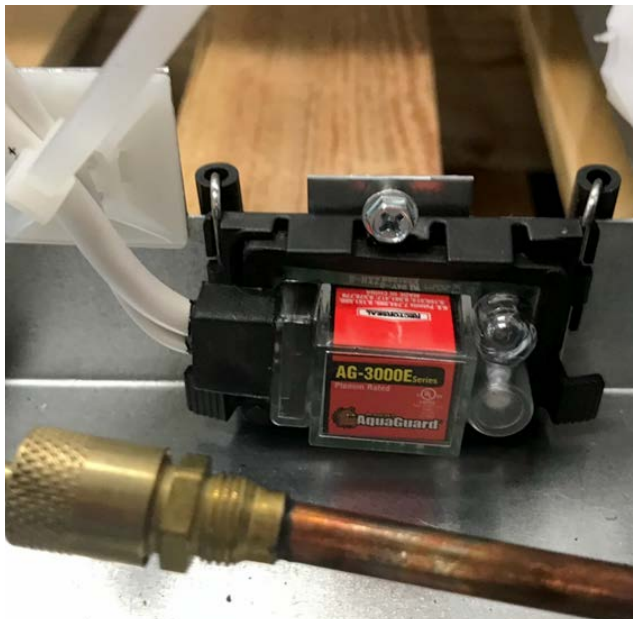
Moisture sensor installed
