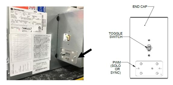
Figure 1 – PWM Installed in Enclosure (example installation location)
