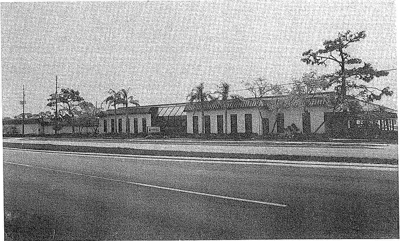
Pictured above is ETI's modern 185,000 square foot engineering center and general manufacturing facility located at 6750 Bryan Dairy Rd., Largo, Florida 34647.
